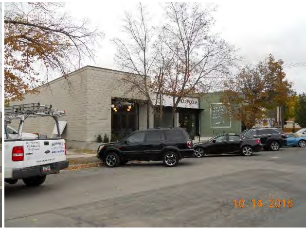
Northwest view of abutting commercial corner
